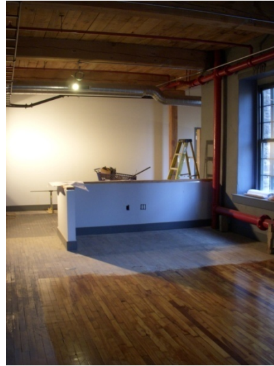
Original view from mid-office toward original door location (since moved). Mid process photo shows bookkeeping half wall, finished floor pre-carpeting.
